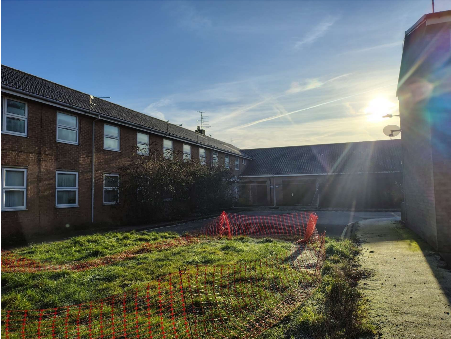
Site Photograph Willow House As viewed from Northwest
